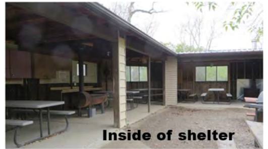
Cook Shelter at Nancy Rutt Tenting Site
